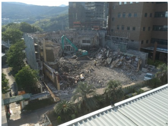
Demolition of the Sojo International Learning Center
